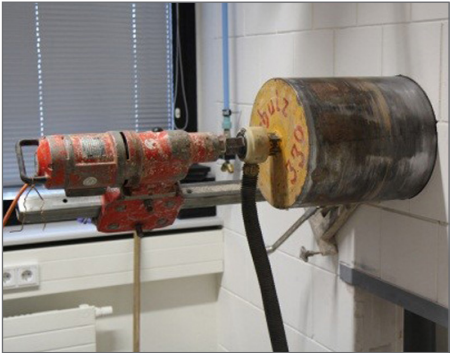
Fig. 2 – core hole drilling
