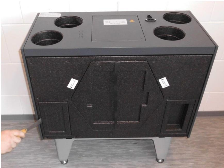
5. Pull the fan with a pliers out of the device.
