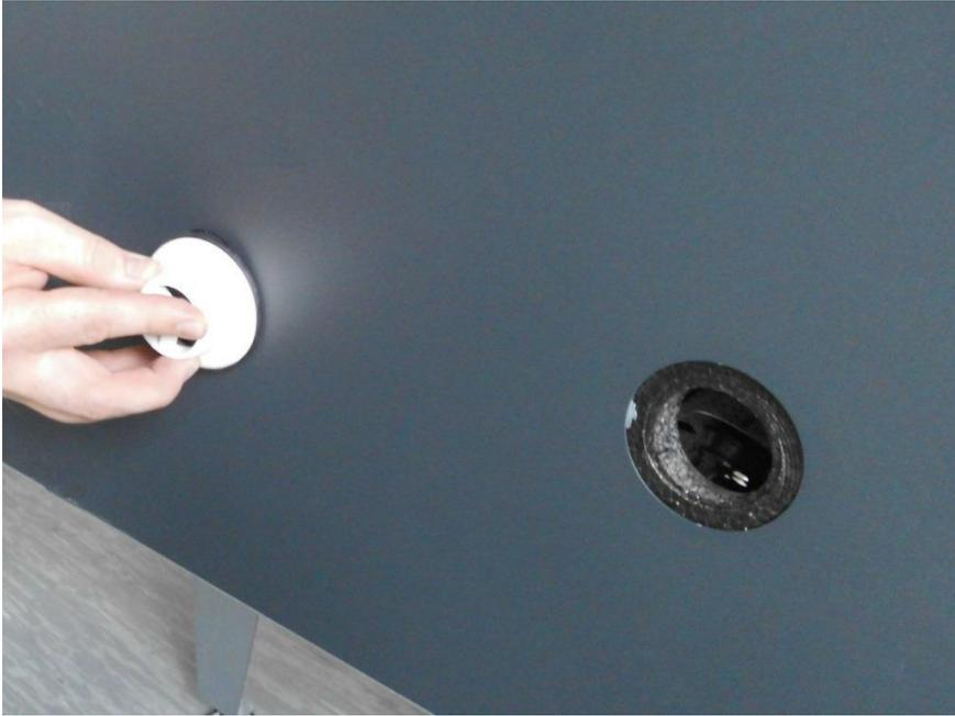
6. Remove the excess sealant.
