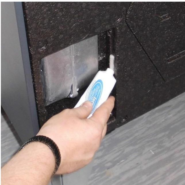
15. Insert the EPP fan cover into the ventilation device and remove the excess sealant
